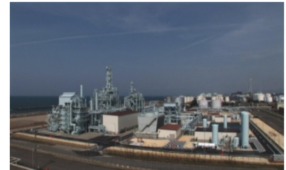
“Japan GTL” Demonstration Plant in Niigata, Japan
