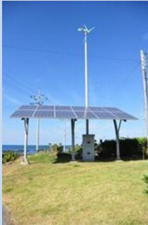
Figure 6-6: Wind-Solar PV Hybrid System in Korea
