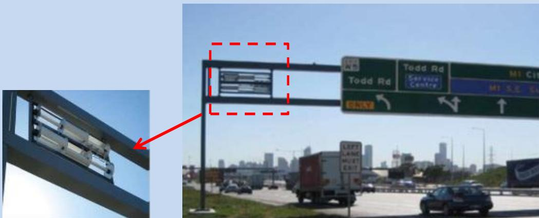
Figure 6-8: Windpods integrated directly to signage in Australia<sup>51</sup>
