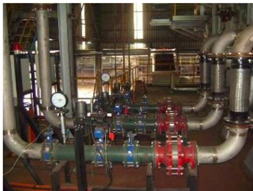
**Figure 5-4: Biogas burners installed at biomass boiler**
