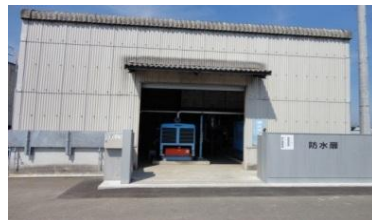
Pump with the waterproof door
