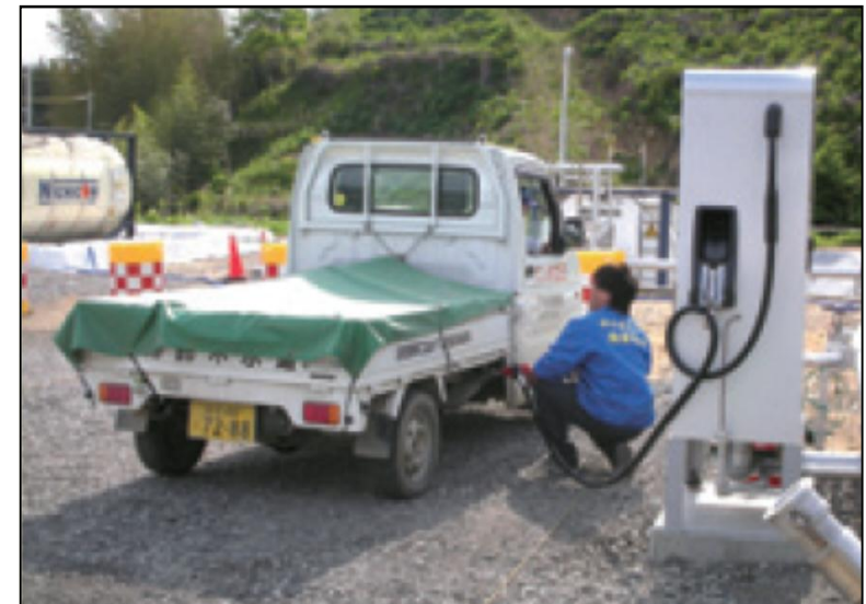
Temporary service station utilizing ISO tank containers
