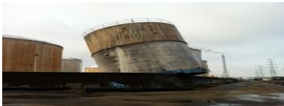
Damage on oil refineries
