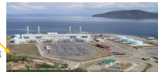
1,200 MW Ilijan Power Plant NPC IPP(KEPCO)
