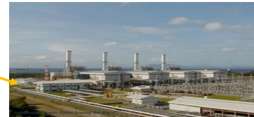
1,000 MW Sta. Rita First Gen/ IPP
