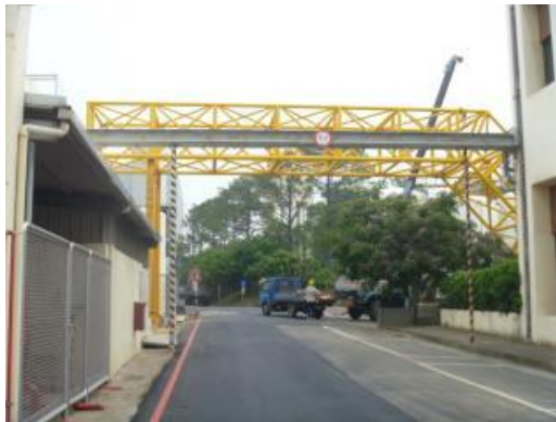
Piping (@ B15 + B17)
