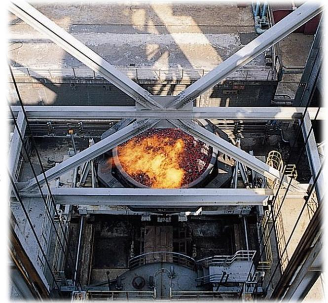
Coke Dry Quenching (CDQ) facility in operation at Pohang steelworks. The CDQ recovers the heat from the hot coke which is converted into electricity. Last year, approx. 140,000 tCO<sub>2</sub> was reduced via the CDQ. CDQs have been installed in all coke ovens except for one which is to be revamped by 2023.
