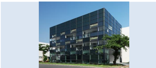
<Side wall> reference: https://www.taisei.co.jp/about_us/wn/2014/140616_3948.html (大成建設HP)
