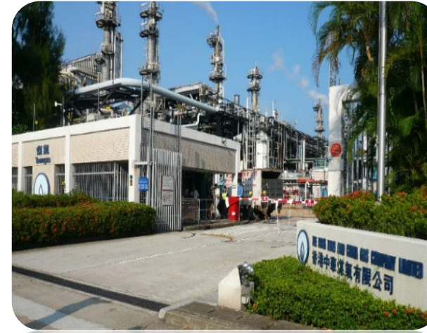
Towngas Production Plant
